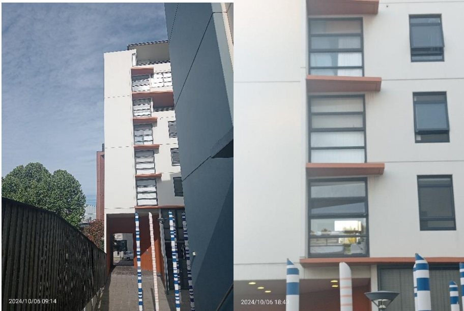
Figure 3 Linc North living areas adjacent to fence line
